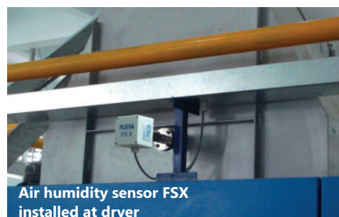
Air humidity sensor FSX installed in exit tube
