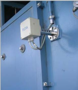
Fig. 2: FS 91 Exhaust Humidity Sensor
