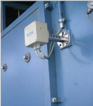
Fig. 2: FS 91 Exhaust Humidity Sensor
