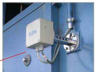
Maintenance free sensor to measure the exhaust air humidity and to control the exhaust fan automatically by frequency inverter.
