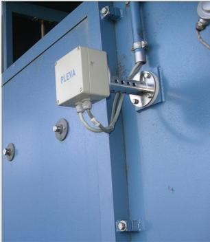
Fig. 3: FS91 exhaust humidity sensor
